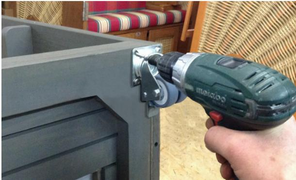
**It is necessary to pre-drill holes with 3mm drill to avoid cracks on wood.** Lockable castors should be fixed on front corners of beach chair.
